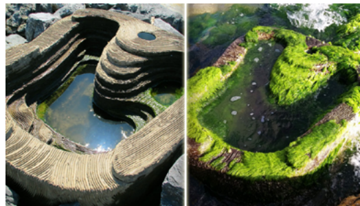
Figure 3. Tidepool Armor, minutes after installation (left); and after 12 months (right).
