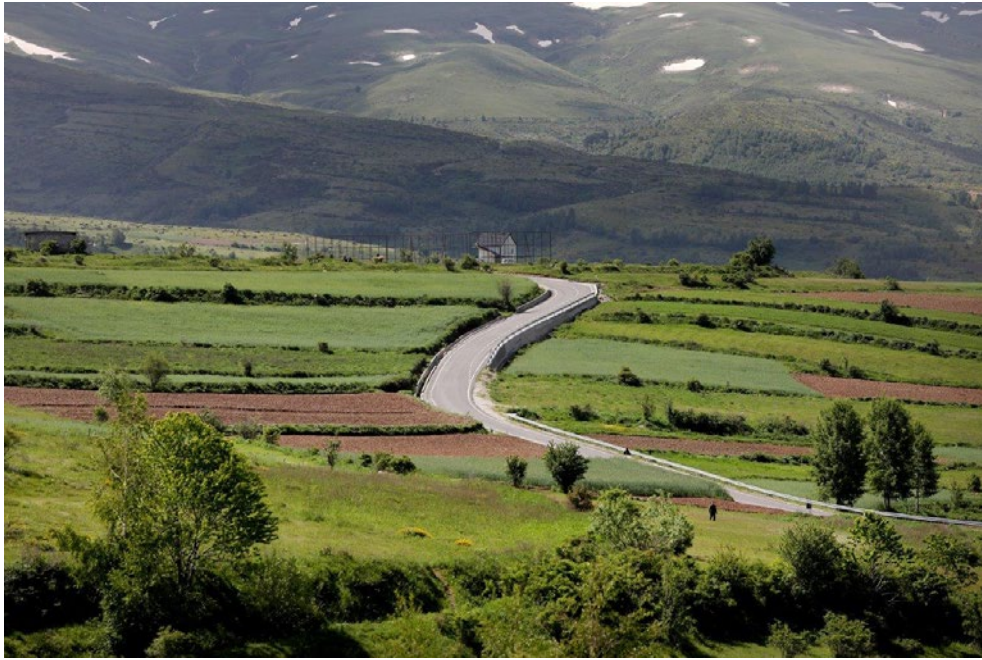
EU support to road maintenance policy in Albania
