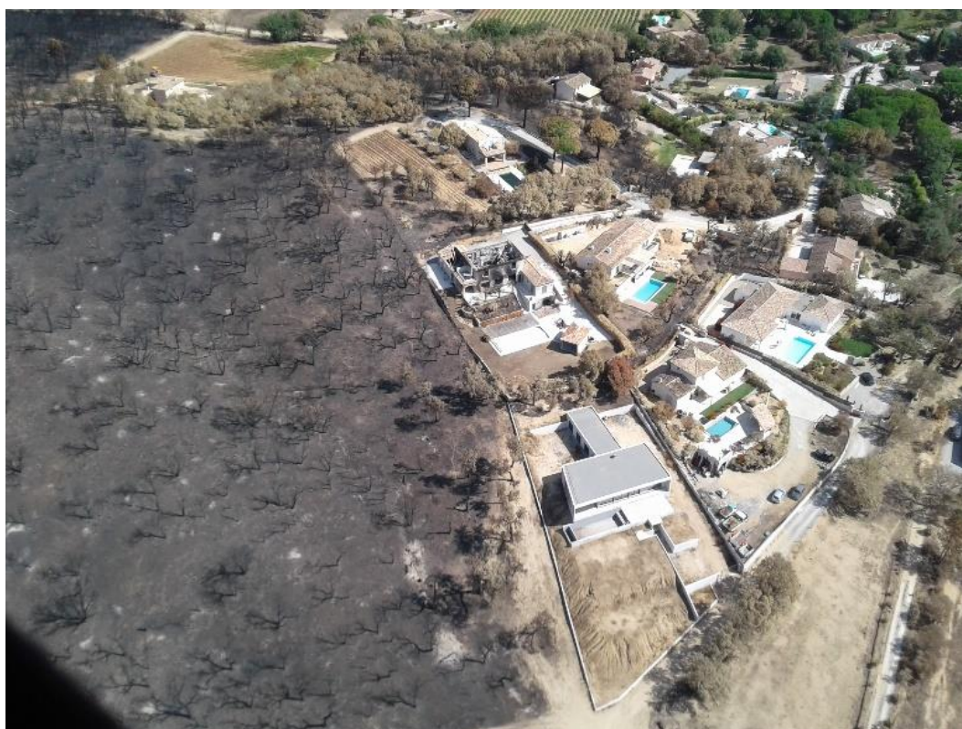
Figure 28. Aerial view of buildings affected.
